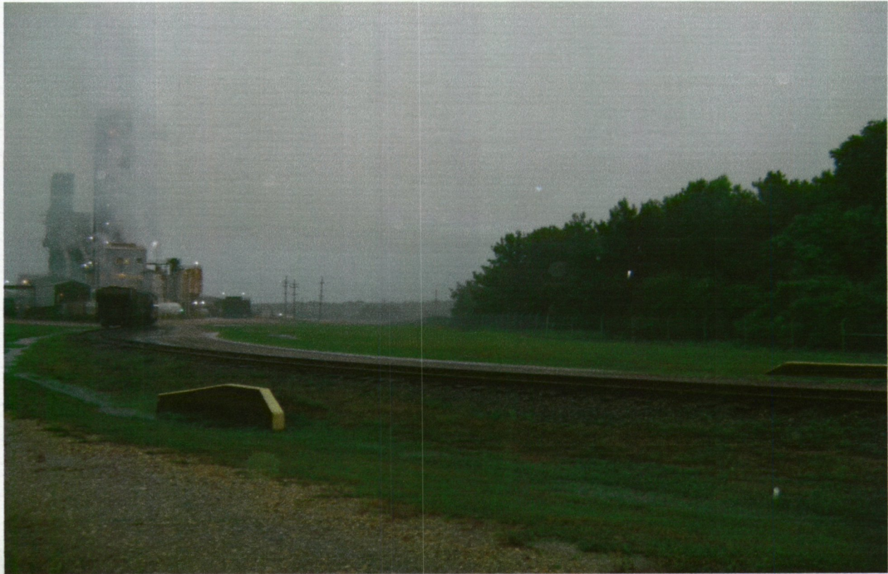
Figure 3. Discharge point at the end of new underground line that collects water from areas in figure 1 and 2 and flows to the head wall under the tracks and into the new line east to Lake Lee (Day Pond). Drain boxes have been installed along the line to capture all of the water on the south side of the road that previously discharged through Outfall 007. View from northwest to southeast.
